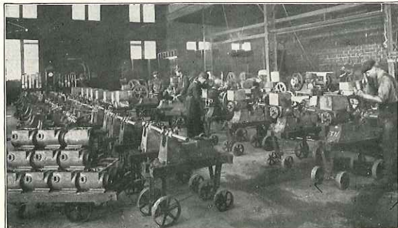
Putting the engines together. Every part fits without any changes.
